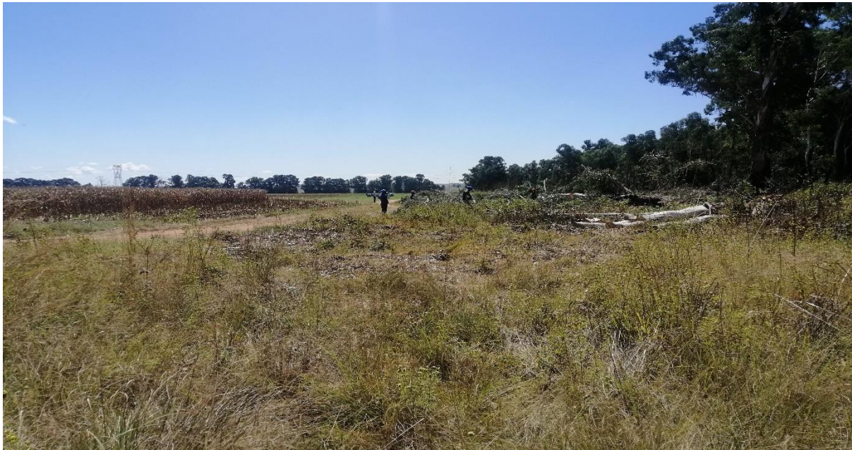
Figure 3: Bush clearing activity in the Eskom powerline servitude.
